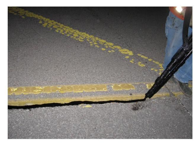
**Crack Sealing Process**
